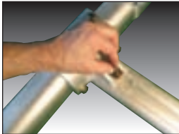
9B T-Bolts inserted
